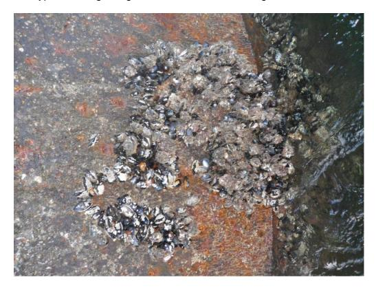
Figure 5: Fouling of mussels and barnacles on central stanchion of bridge.
