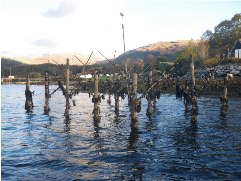
Figure 10: Sections of old pier at Creran Moorings.
