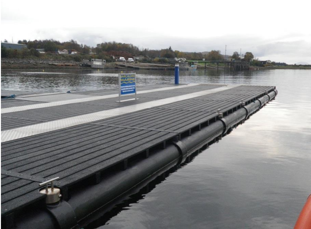
Figure 20: Pontoon at Marine Resource Centre.
