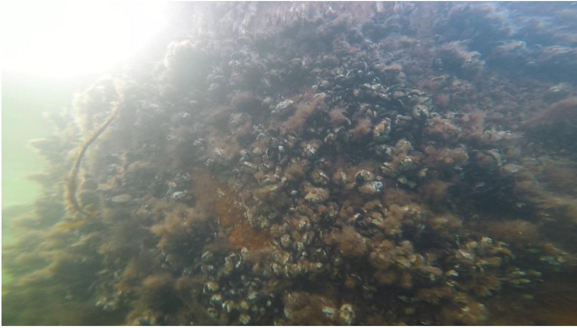
Figure 28: Video footage still of bridge stanchion.
