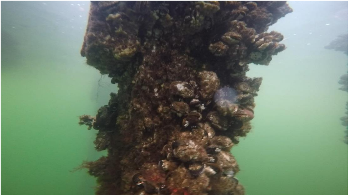
Figure 26: Video footage still of pier stanchion.
