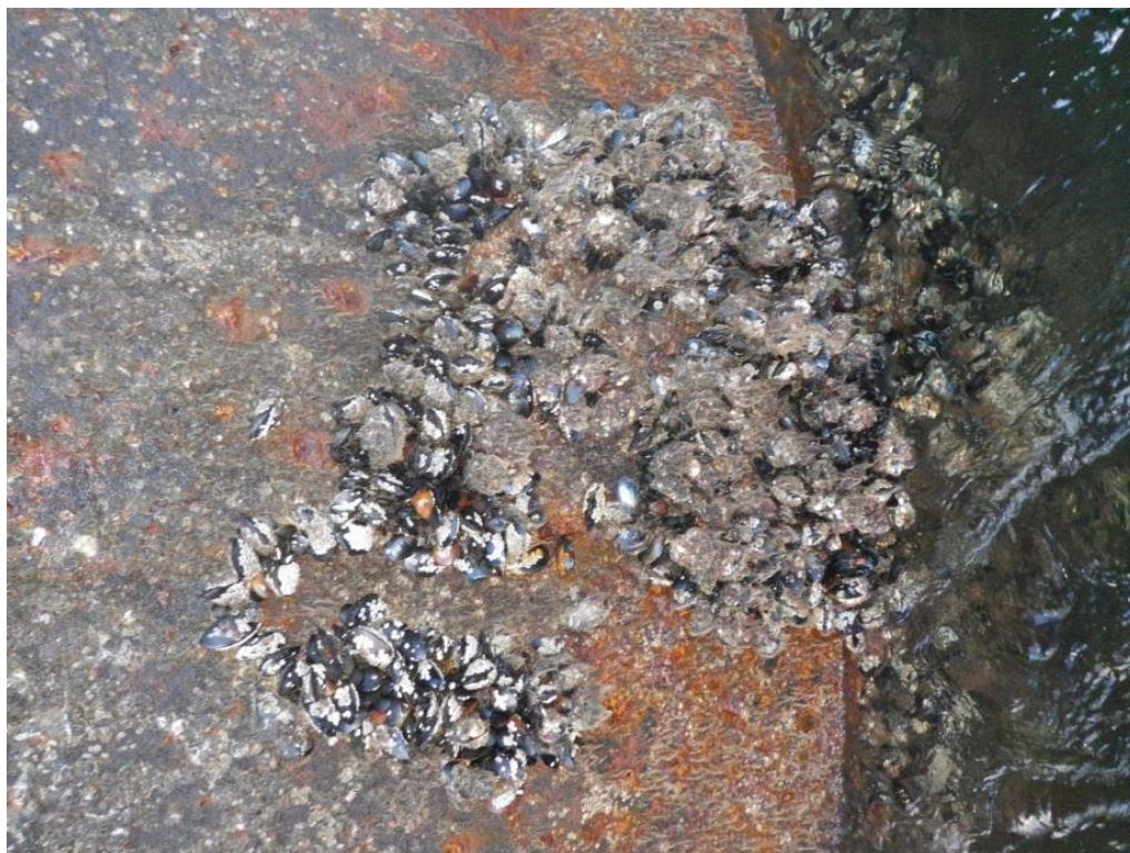
Figure 5: Fouling of mussels and barnacles on central stanchion of bridge.
