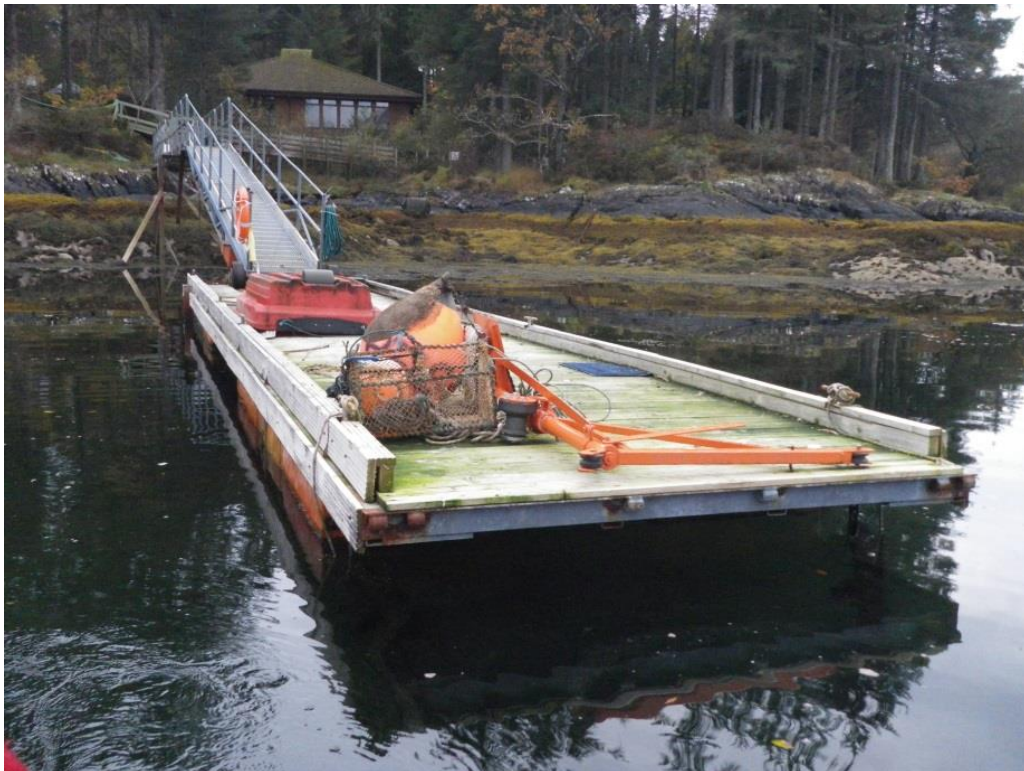
Figure 19: Pontoon at Sealife Centre.
