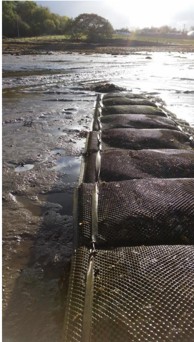
Figure 3.12: Sighting along Dry Trestle.
