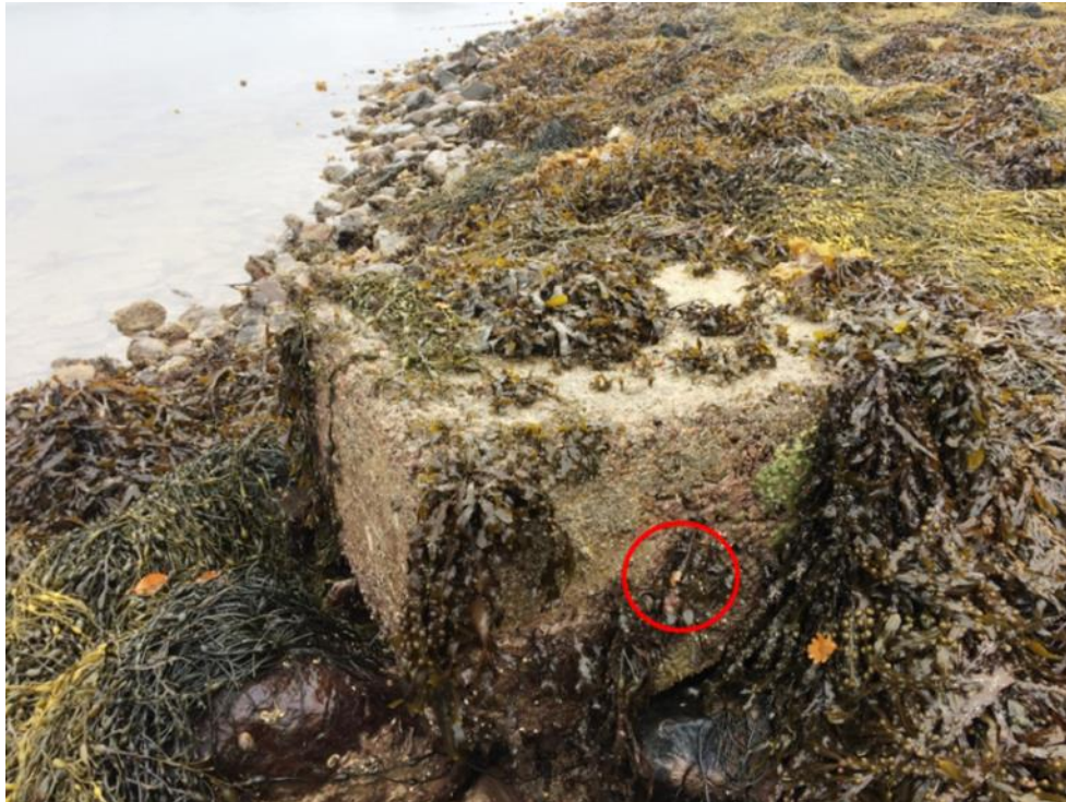
Figure 4.3: Location of suspect sample on the concrete block (red circle).
